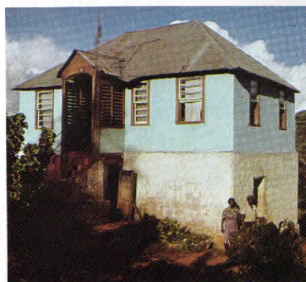
Lime washed walls with 'red work'.
