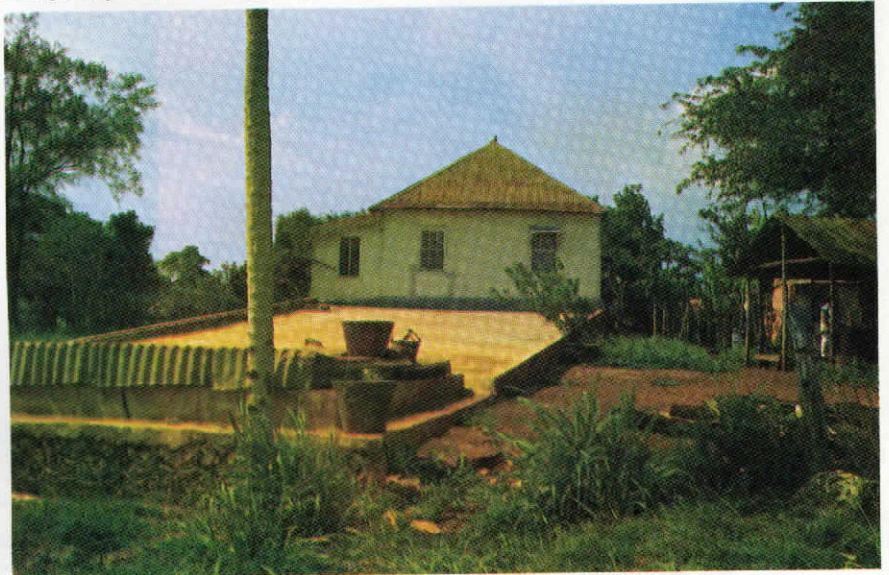
Water catchment with water tank of kick and buck in the foreground, St. Elizabeth.
