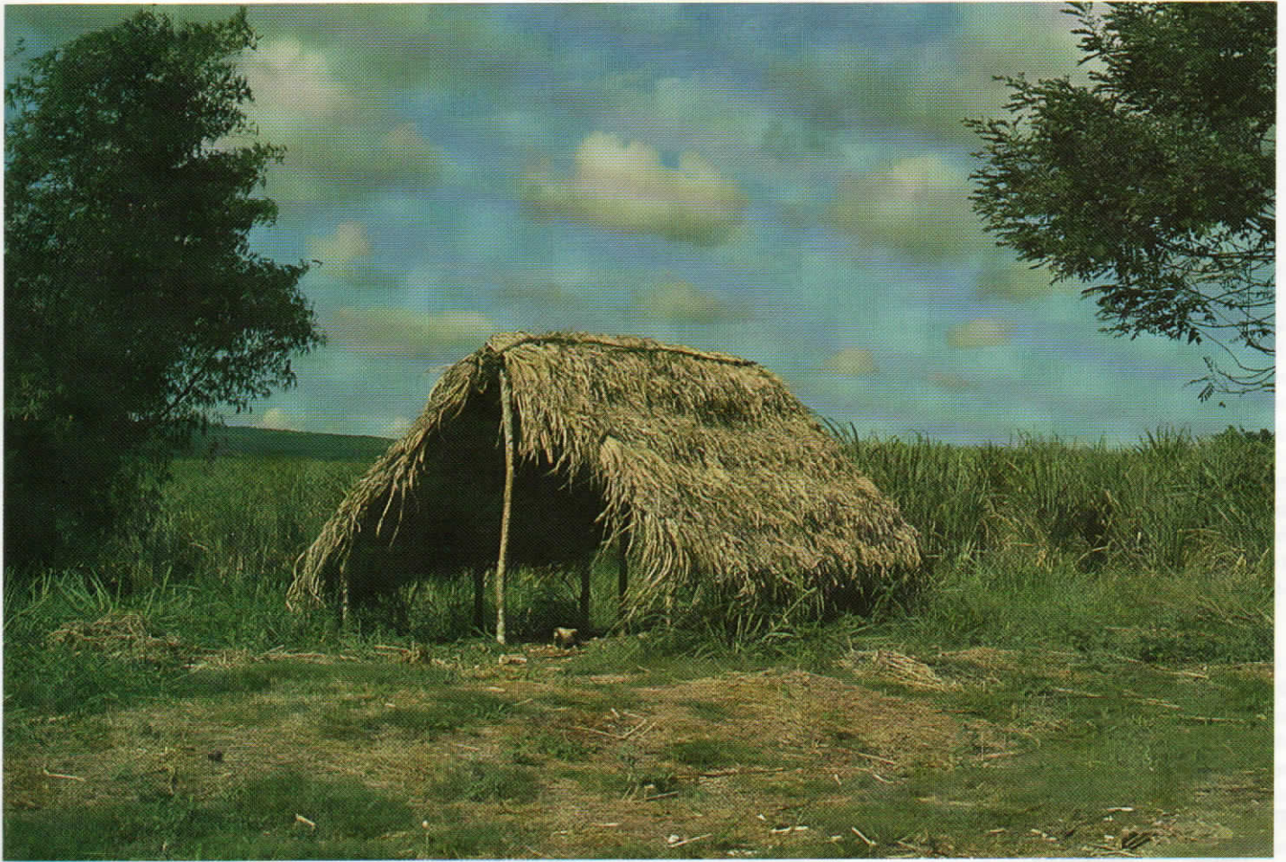
Shelter thatched with cane tops, Hanover.
