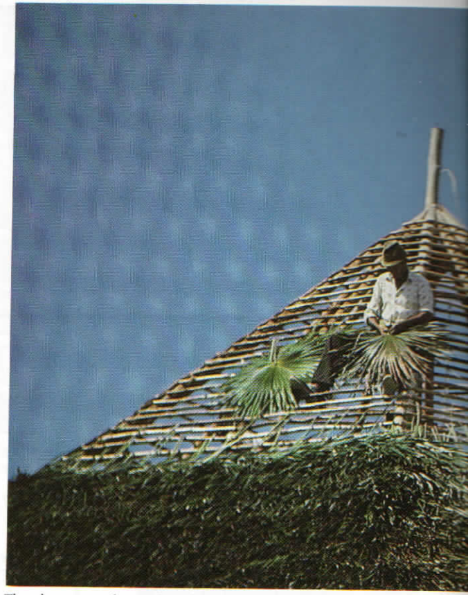
Thatchers at work on a Negril restaurant using Silver Thatch.
