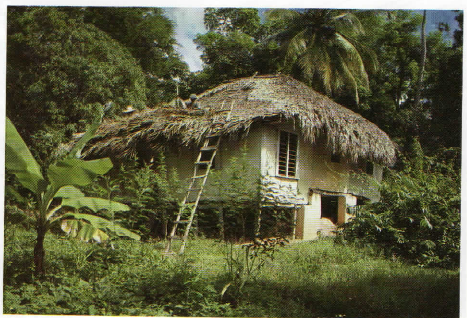
Thatchers at work repairing a roof in St Elizabeth.
